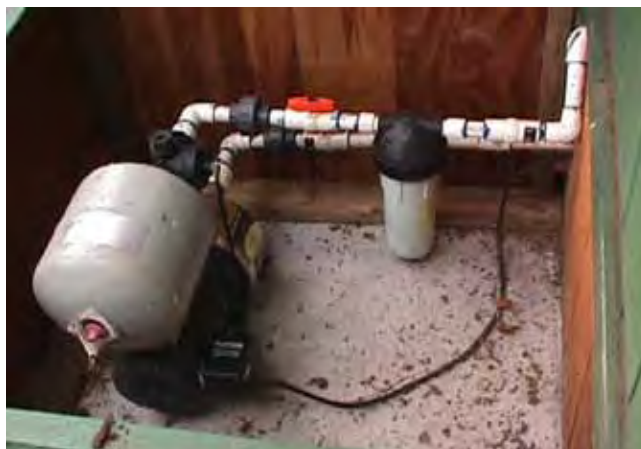
A small but typical electric pump. The pump sits below a pressure chamber. A coarse filter hanging from the inlet pipe filters the water before it enters the house.
